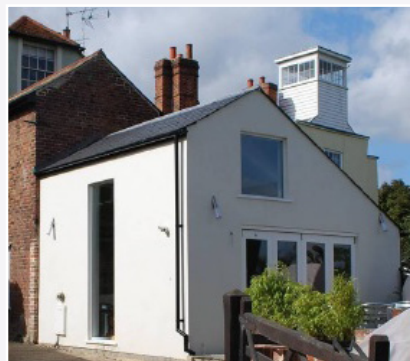
Extension to historic building – Winner of Maldon District Conservation and Design Award 2011 for Design
