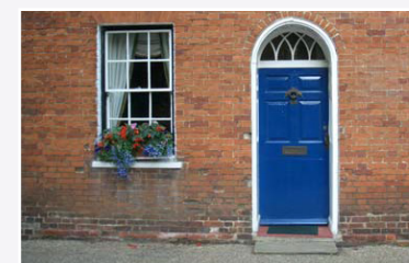
Brick and window detail, Bradwell on Sea
