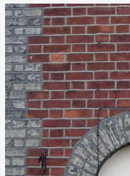
Typical details: red brick with quoins of gault brick, Heybridge Basin
