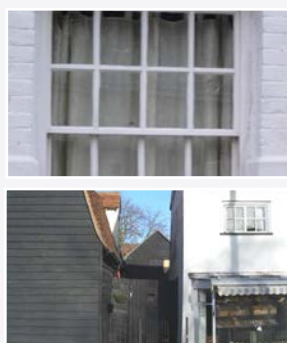
Typical details: vertical sliding timber sash windows, Heybridge Basin and weatherboarded cottage, Goldhanger
