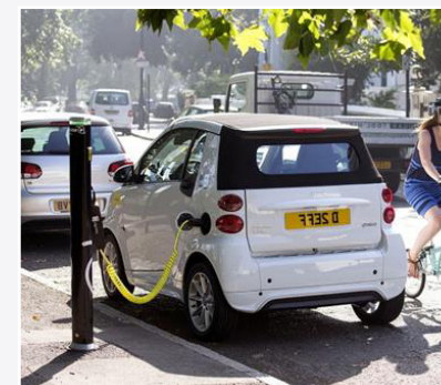
Electric charging point
