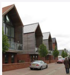
Roof overhangs providing protection to glazed facade
