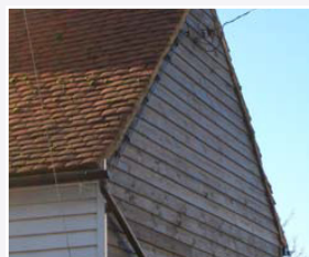
Typical details: steep plain tile roof, with weatherboard painted white. Tillingham
