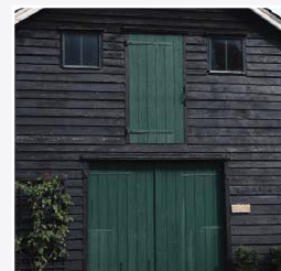
Weatherboard - a classic building material used throughout East Anglia in particular Essex. This style has been adopted for many new houses which helps them to blend in with older buildings in the area
