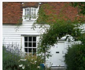
Typical details: weather-board, tiled gambrel roof, Bradwell-on-Sea
